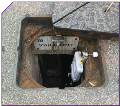
An Integrated Sensor Module and Ubiquitous Wireless Network for Smart Drainage System 結合無線傳感模組及網絡的智能渠道管理系統
