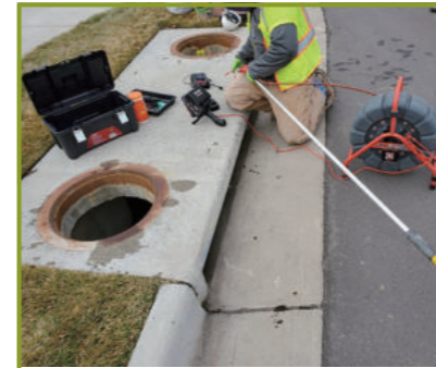
Video Analytics Based Detection of Defective Underground Stormwater Drains 應用視頻分析技術以檢測地下雨水渠異常情況
