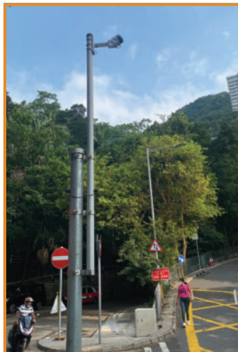
Real-time Vehicle-actuated Traffic Signal System 應用於改善交通流量的車輛偵測及警報系統
